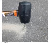
Remove dust from holes. Insert the nylon plugs (supplied) and tap flush with road surface.
