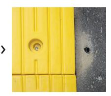
3. Move the modules aside and drill out the pilot holes with a 14mm masonry bit.
