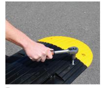
6. Wind in fixings securely using socket wrench or impact driver.
