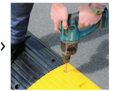
2. Pilot drill the mounting holes using a 10mm masonry drill bit.
