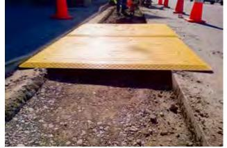
Safe Covers offer a safe, slip-resistant passage through footpath works for pedestrians and small vehicles like motor scooters.
