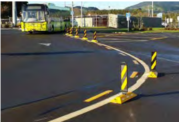
Traffic Separator Pods offer additional lane separation on top of a painted line.
