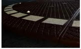
Reflective panels and cat's eyes make the Rubber Roundabout visible in darker conditions.
