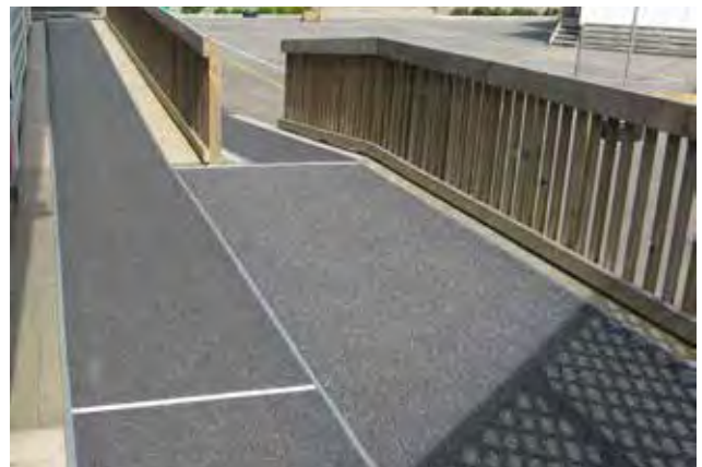
Use on timber ramps and decks to prevent slips.
