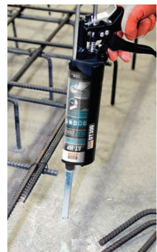
Rebar Doweling
