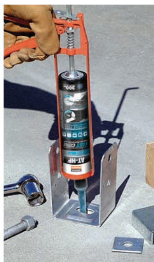
Threaded Rod Anchoring
