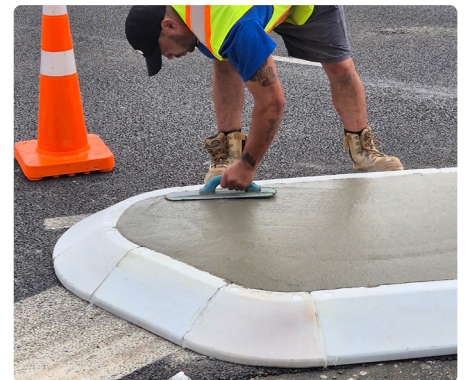
▲ Smooth and finish concrete
