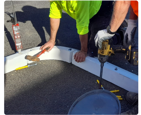
▲ Drill fixing holes; secure blocks with screws
