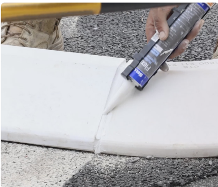
▲ Seal gaps between blocks
