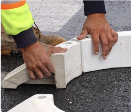
▲ Position blocks according to plan
