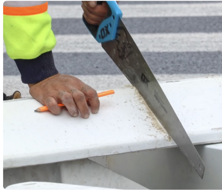
▲ Mark and cut kerb blocks to fit
